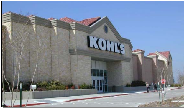
Illustration 10-12 EXAMPLE OF FAÇADE ARTICULATION
