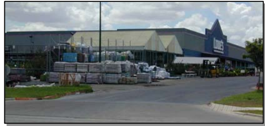
Illustration 10-12 AN OPEN STORAGE AREA IN NEED OF SCREENING
