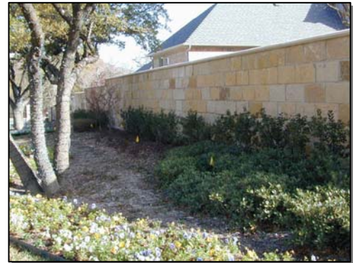
Illustration 10-5 MASONRY SCREENING WALL
