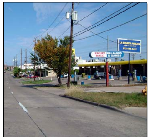
Illustration 10-16 EXAMPLE OF THE RESULT OF A LACK OF SHARED DRIVEWAYS & CROSS ACCESS
